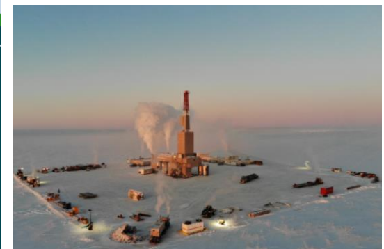
Drilling rig on location
