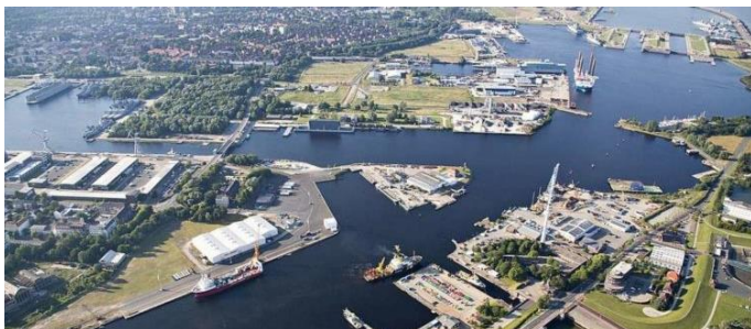
Access to key energy hub Wilhelmshaven, Germany
